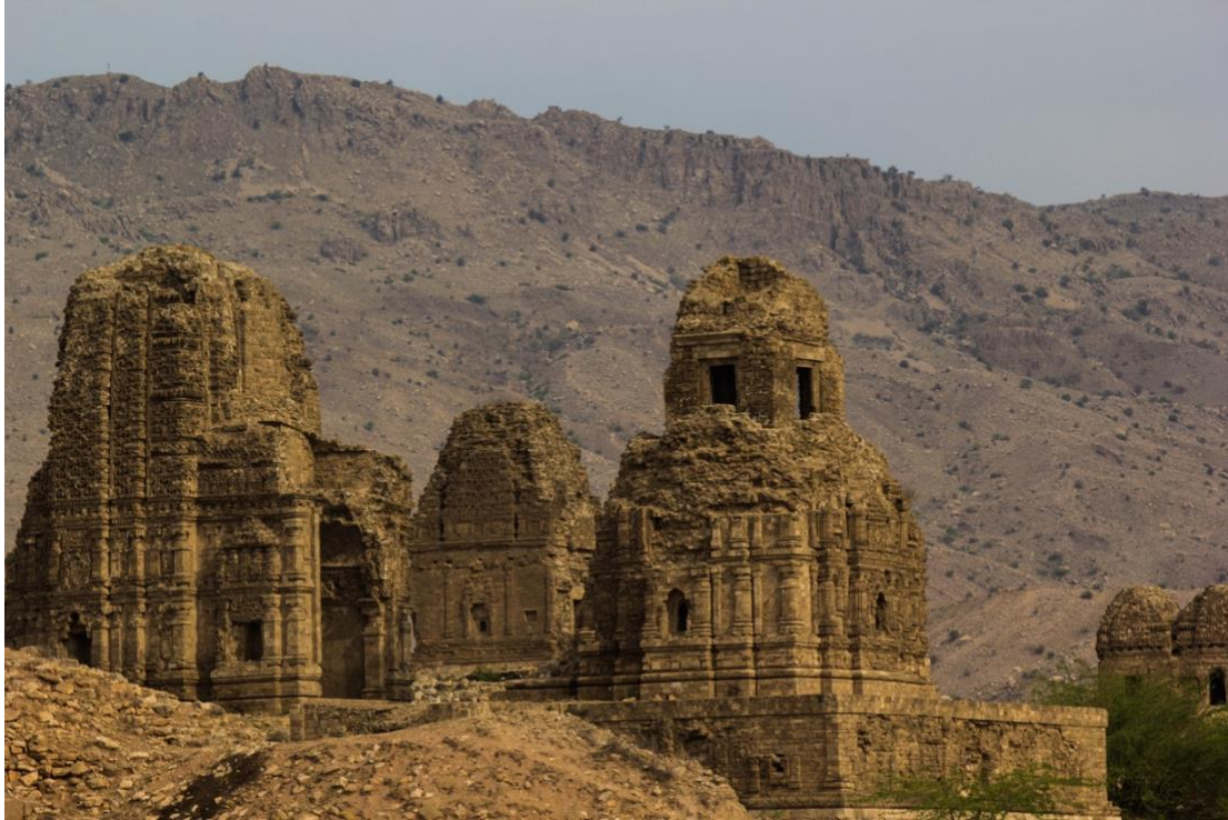
Figure 1. Bilot, Temples B (right), C (left), and D (centre), with Temples F and G in the distance (right), from south-east. (Photo courtesy of Adam Hardy, with thanks to Zeeshan Ghani and Samra Khan)
